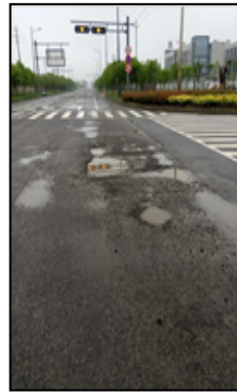
Pothole Inspection
